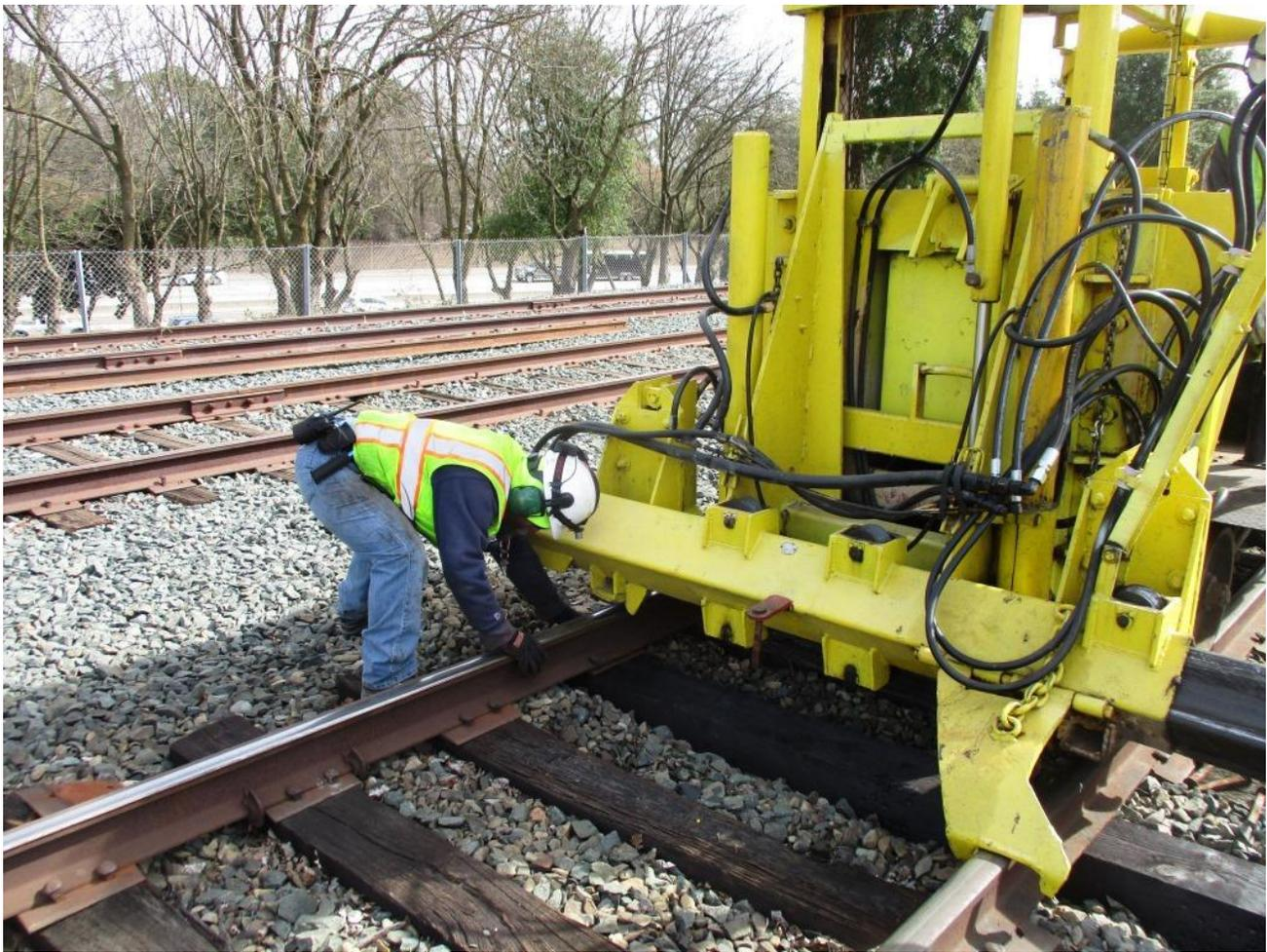
With the 125's track-jacking system lifting the rails slightly, Joe is able to squeeze a tie-plate between the tie and base of the rail
