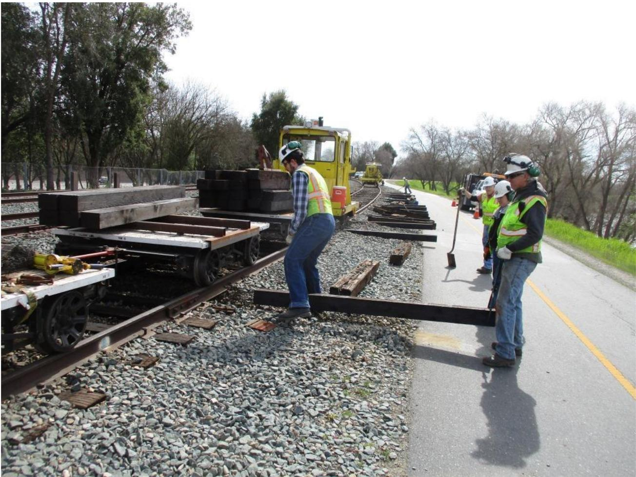
Weston and Steve then line the new ties up with the empty cribs for the 125 to pull in
