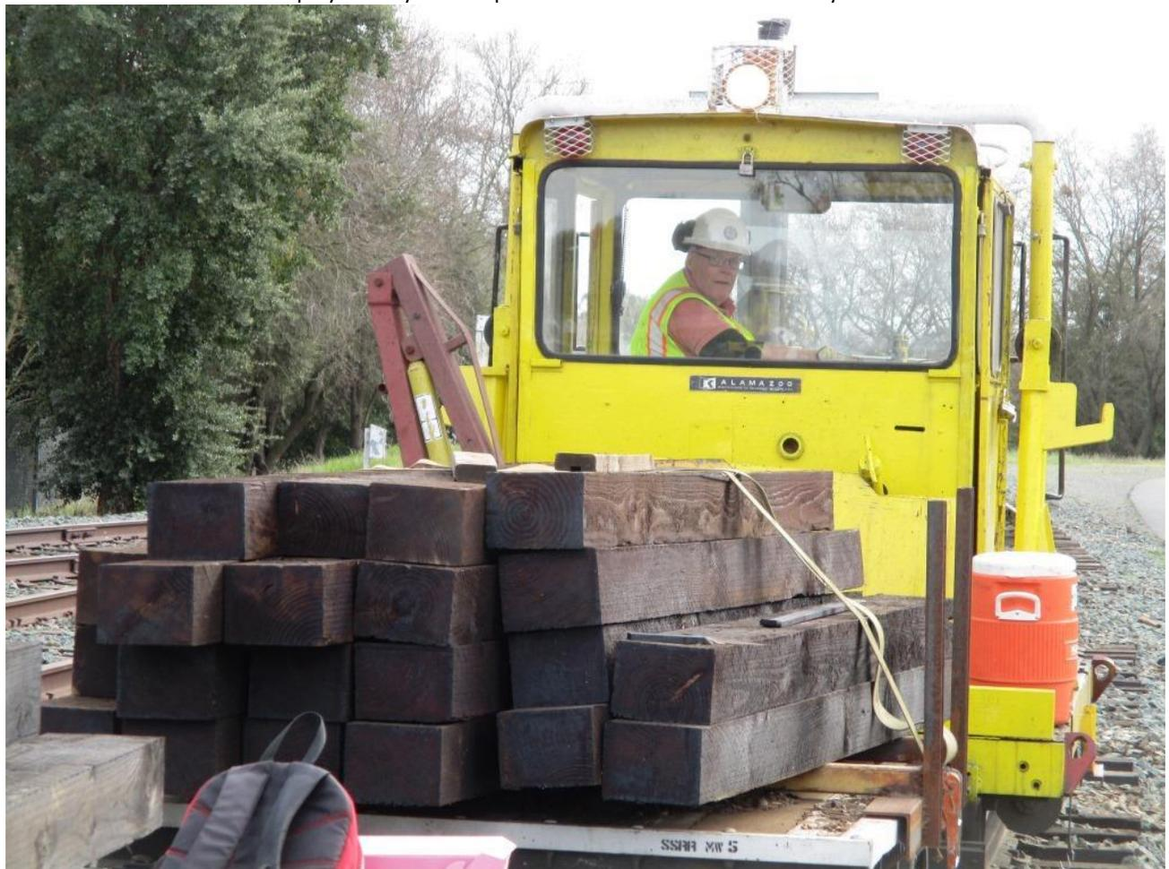
As spiking work progress north, Bill moves the Kalamazoo which was shoving the flatcar with the hydraulic power unit
